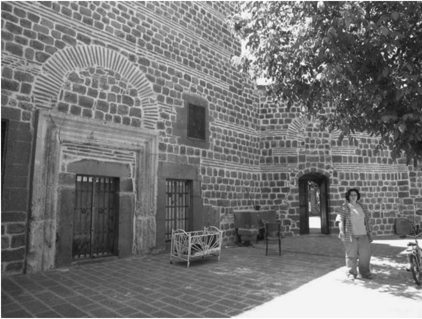
Fig. 2.4.5 Wall of the sanctuary part of the Church of Yoldath Aloho
